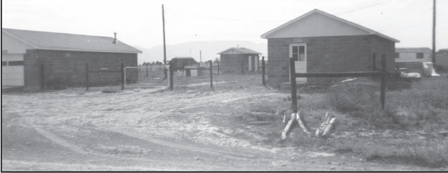
The Machine shop, left, Woodshop, right, and Mabel I house in the background, as they appeared in February 1963. Both shop buildings were expanded with additions later.
